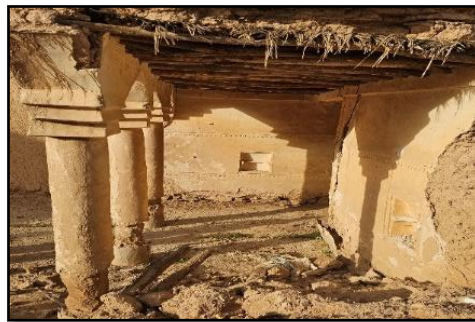
Figure (5) The portico of the Al-Tuwaijri house in Majma'ah (photographed by the researcher)
